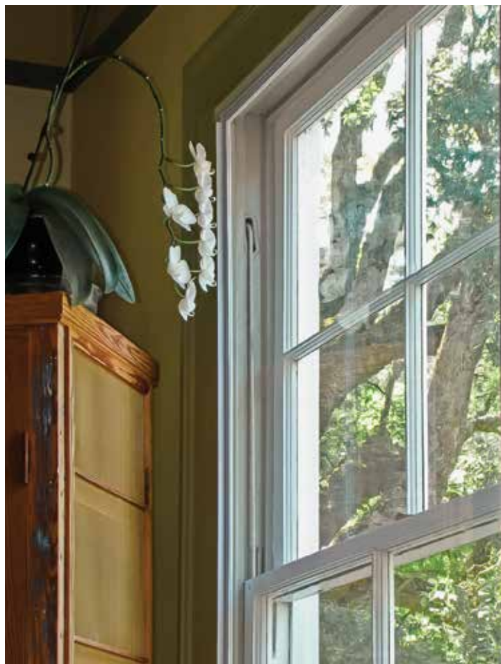
ABOVE Nearly invisible, an Innerglass window fits tightly inside the inner frame of a double-hung window, creating a sound and air buffer. Installing the windows on the inside also prevents condensation. RIGHT Kimber and David Degling have been making interior window inserts for 30 years.
